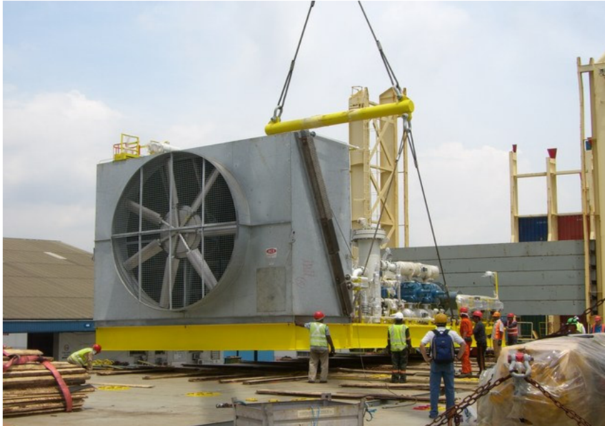
Handling 2 units of Gas Compressor onto Barge Winstar 8
