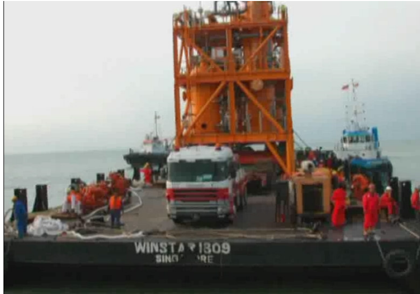
Roll-On and Roll-Off Operation of Gas Module
