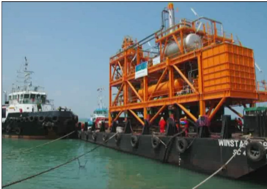
Gas Module mounted on Barge Winstar 1809 which acts as its base
