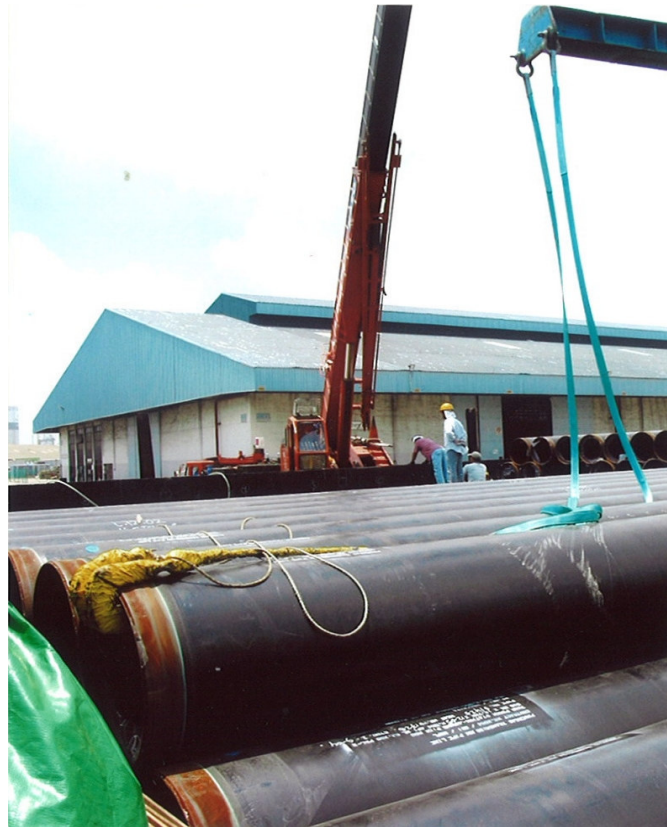
Unloading the Coated Pipes from our Barge in Jurong Port The collection was done in Batam
