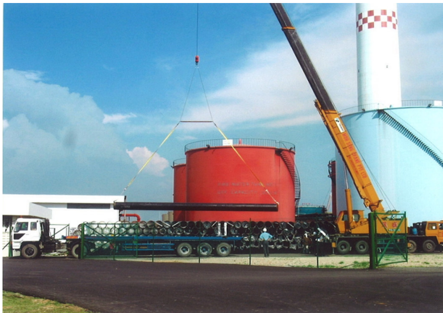
Offloading and Stacking the Coated Pipes in the open storage inside Tuas Power Station
