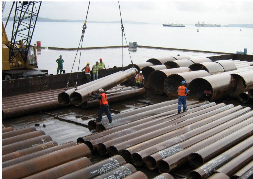
Sea Transportation of these Steel Pipes from Batam to Pasir Gudang done by Winstar Victory
