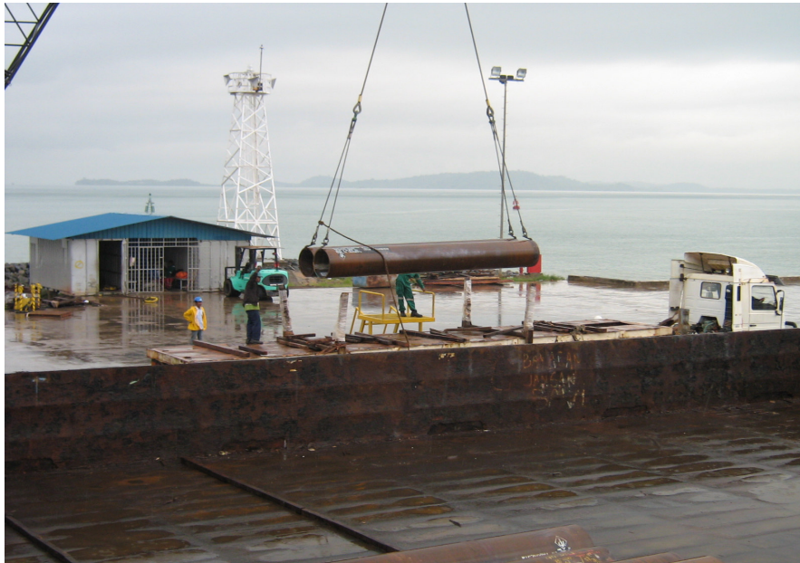
Loading and Stowage of Steel Pipes onto Barge Winstar III
